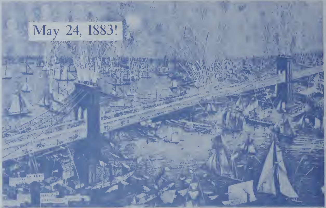
Fireworks, naval and shore batteries, church bells hailed the opening of the bridge. The people of the Cities of New York and Brooklyn took the day off to celebrate.
